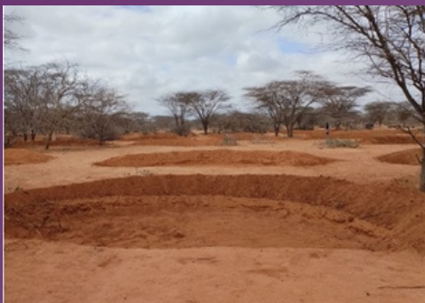
Part of 350 half-moon bunds dug by Balich WRUA facilitated by RAPID+
